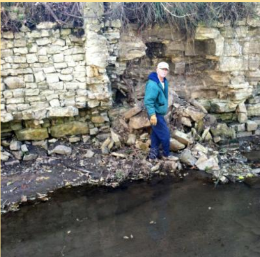
Volunteer Russ Mayer stands in front of 1850s mill ruins eroding from a creek bank near Nebraska City. It is one of Nebraska's earliest water-powered mills. Recent excavations by the NSHS Highway Archeology Program are helping document and preserve the site.
