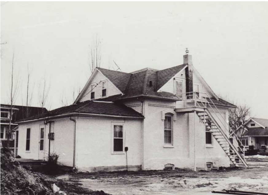
View looking SE showing N & W facades Photo by Troy Lewison, Jan 1986, Star Publishing Company, South Sioux City, NE (NSHS H673.5-4611)
