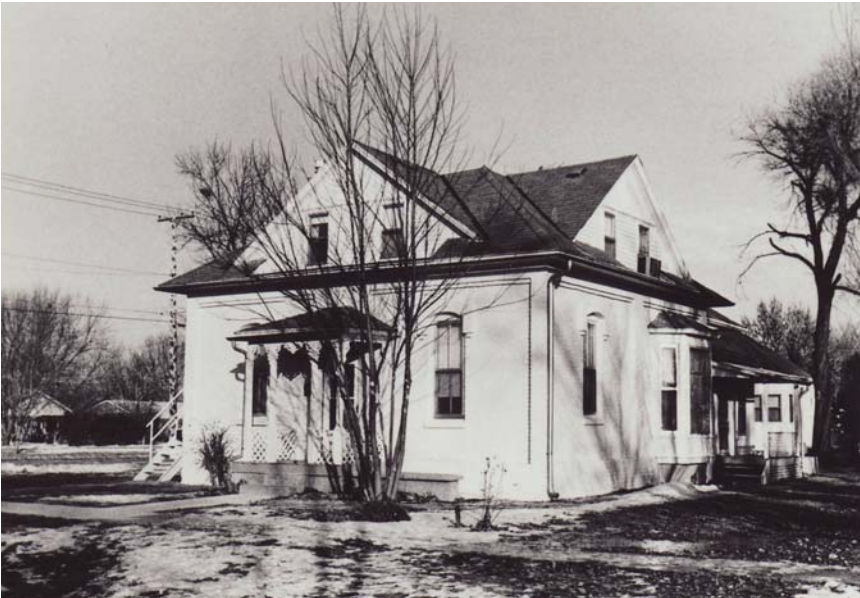
View looking NW showing S (front) & E facades Photo by Troy Lewison, Jan 1986, Star Publishing Company, South Sioux City, NE (NSHS H673.5-4612)
