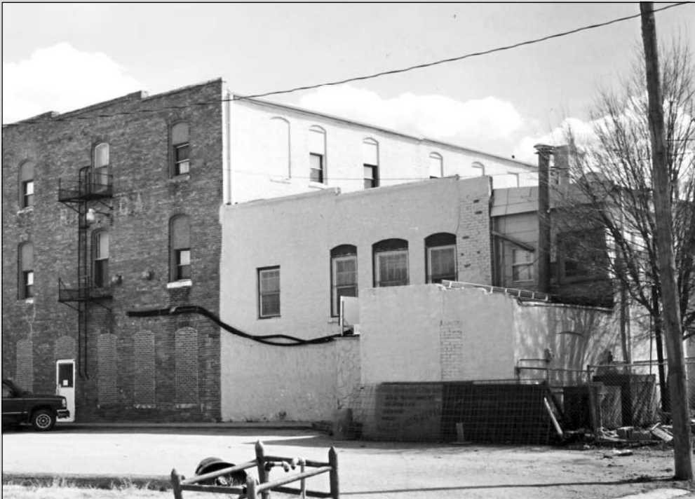
Photo 3 of 7. overview of north façade, view is south-southeast. Photo by Michael Anderson, 2002, Nebraska State Historic Preservation Office
