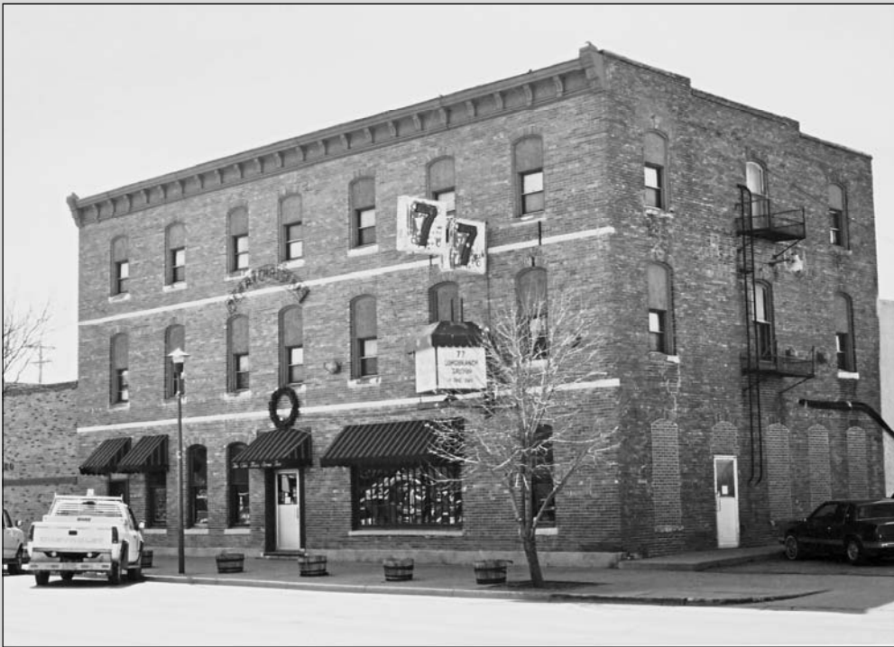
Photo 1 of 7. primary façade, view is west-southwest. Photo by Michael Anderson, 2002, Nebraska State Historic Preservation Office
