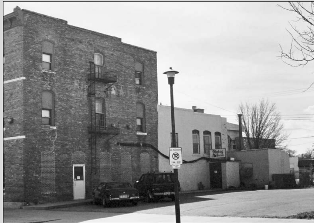
Photo 2 of 7. overview of north façade, view is southwest. Photo by Michael Anderson, 2002, Nebraska State Historic Preservation Office
