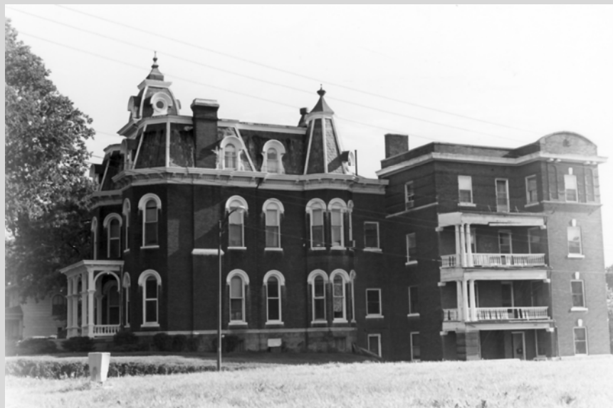
North elevation looking southwest NSHS H673.5-2379
