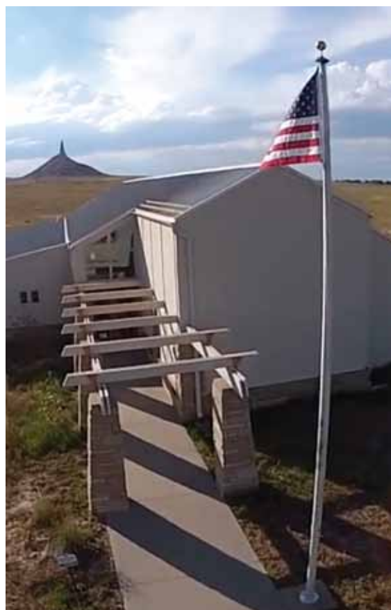
The Ethel S. and Christopher J. Abbott Visitor Center, from a video by David Boff of OutsideOurBubble.com. See nebraskahistory.org/sites/rock
