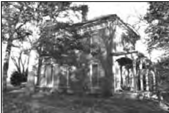
House in Ashland, SD01-009
