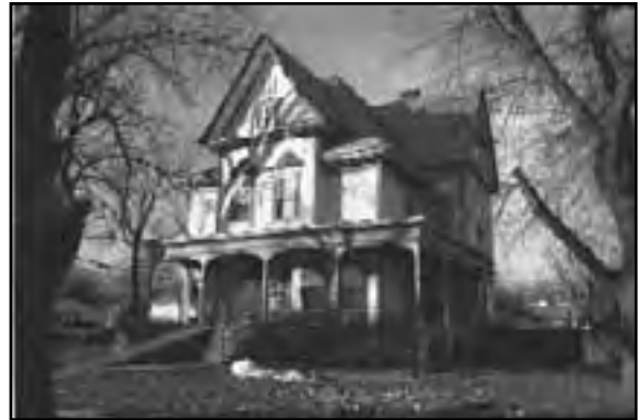
House in Ashland, SD01-051
