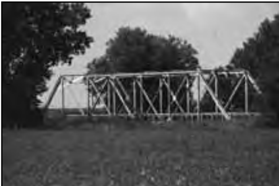
Bridge near Colon, SD00-184
