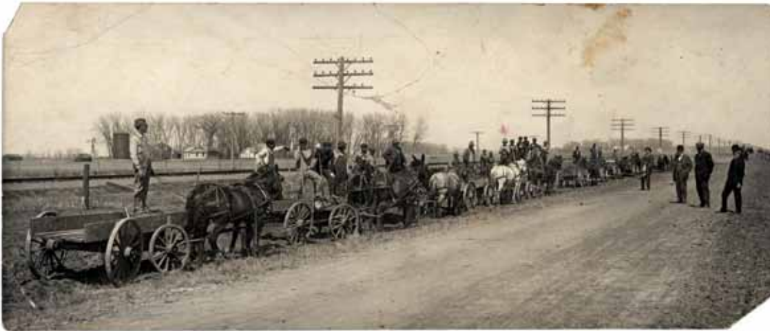
A grading crew works on the Lincoln Highway near Central City, Nebraska, in 1915, the same year the Grand Island Seedling Mile was built to promote concrete pavement. NSHS RG2241-1-70
